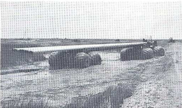
Dredge Pipe Tailing
