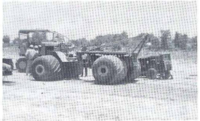
Dredge Pipe Tailing
