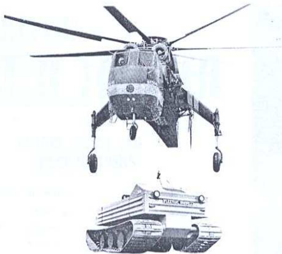
Fully amphibious FN 10 — easily transported by helicopter 1000 lb. payload.
